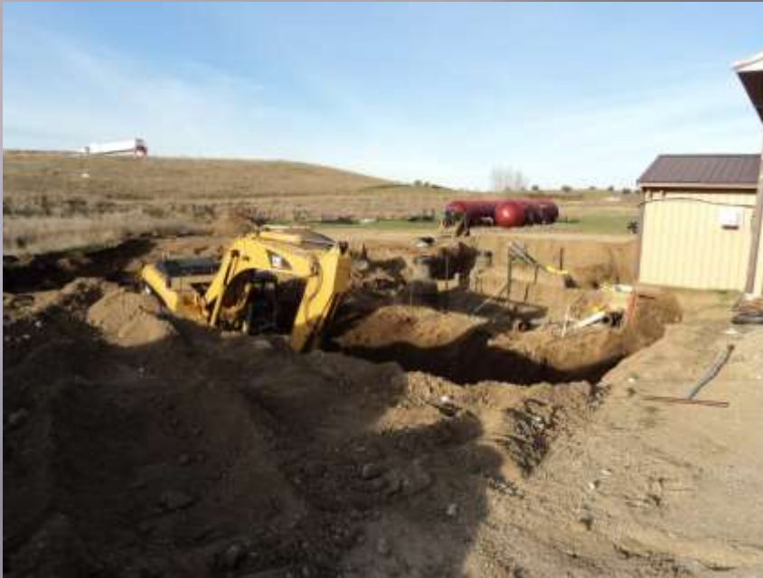
View west of leachate storage tank installation
