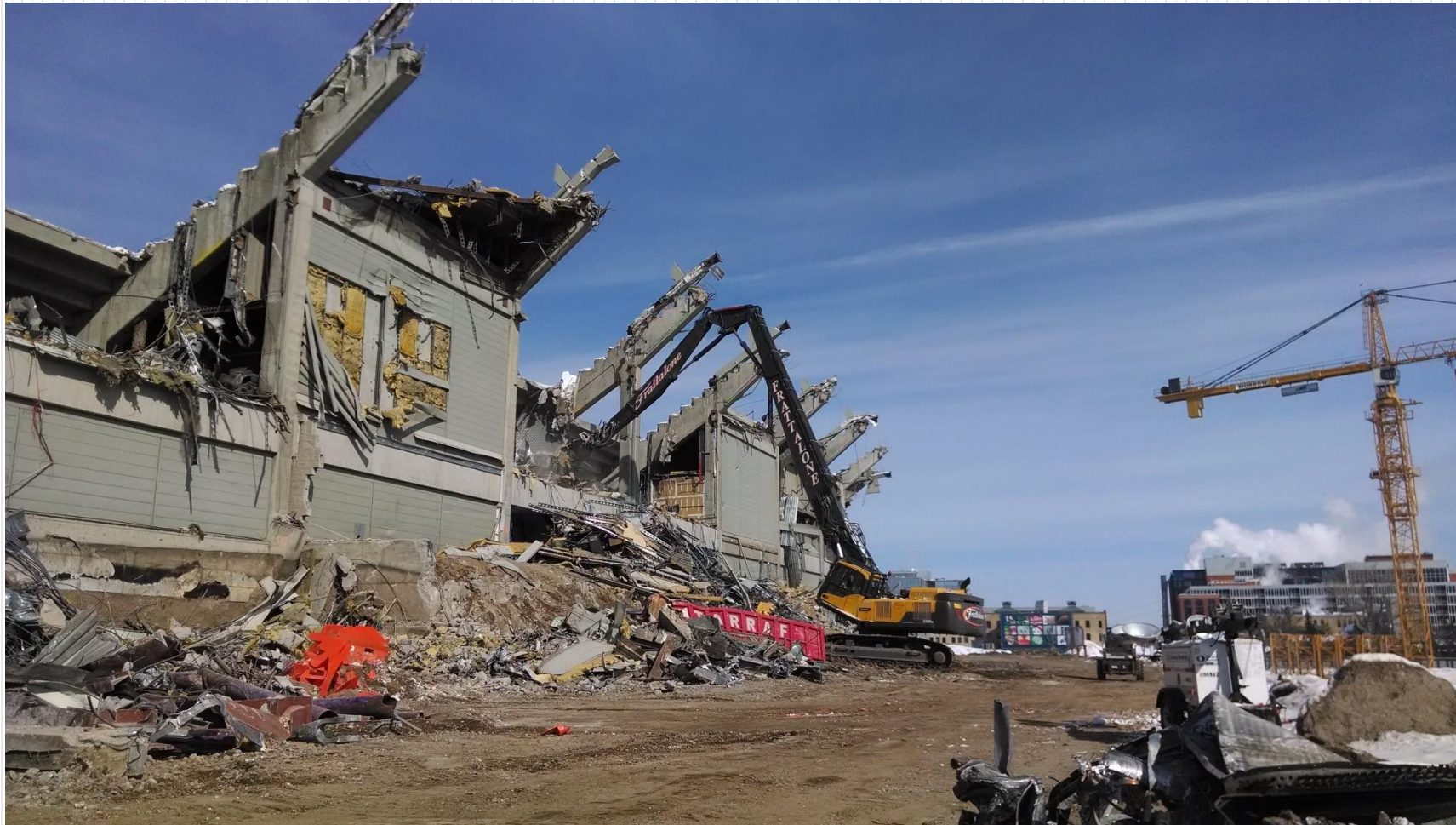
MetroDome Demolition with new Volvo EC480D High Reach Demolition Excavator
